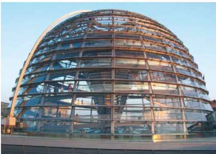
Figure 1. Dome over the Reichstag Building in Berlin, by Sir Norman Foster.
