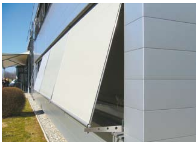
Figure 4. One of the more popular external shading systems: a drop-arm awning
