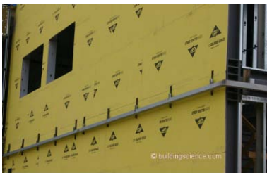
Fig.14 Foto of modern lintel bracket that permits unbroken layer of insulation to pass behind, before the brick wall facing is put up.
