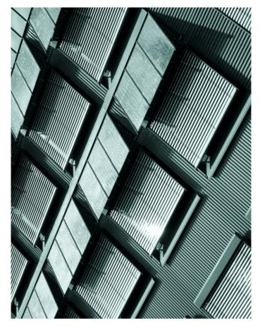
Dynamic shading on glazing can keep more than 90% of the heat outside
